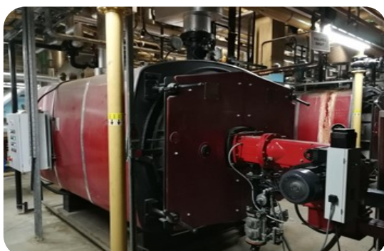
SDH North Boiler Plant (1992 LTHW plant with new modulation burners fitted in 2016)
