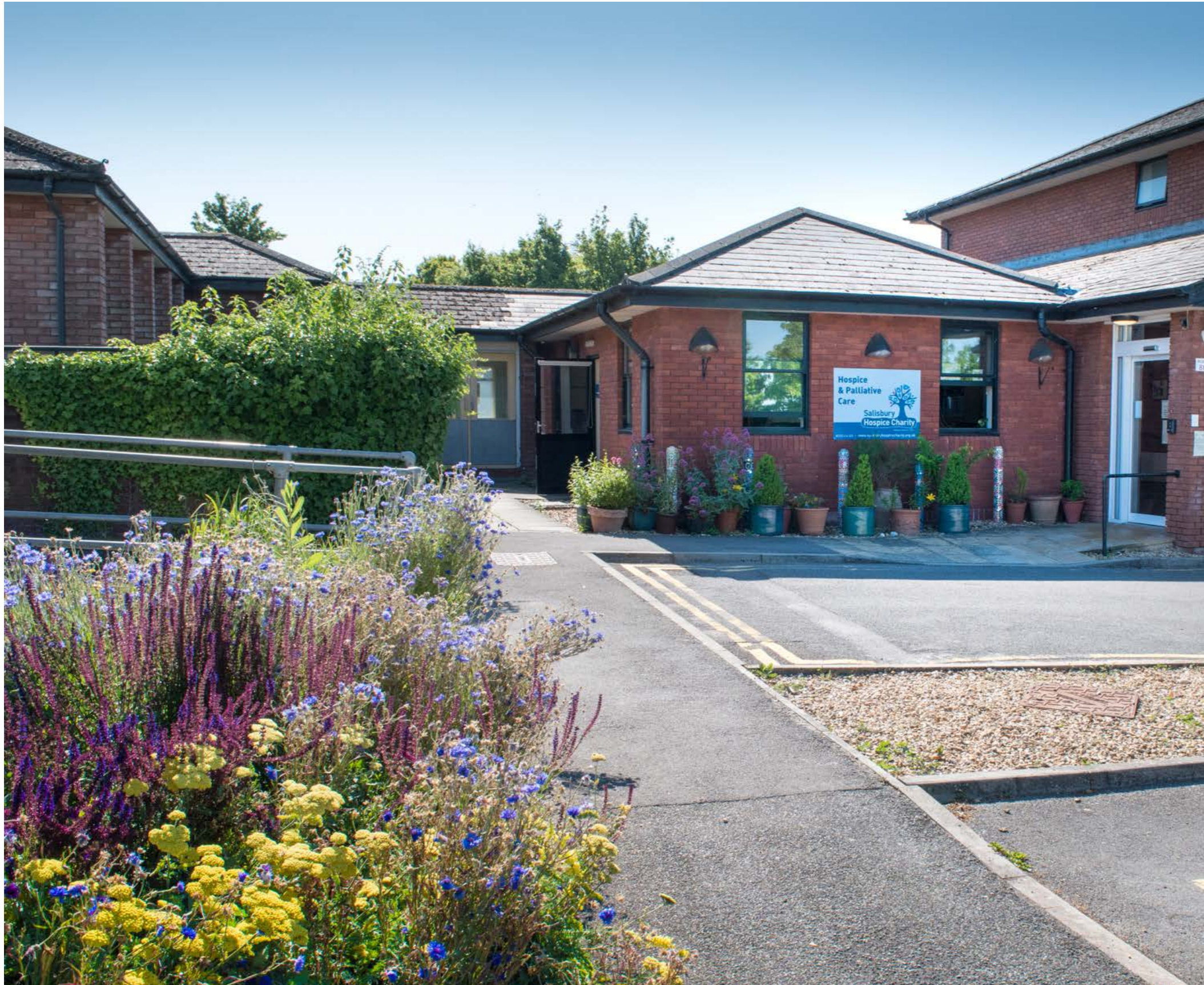
The Hospice car park with disabled parking, pathway leading into Glanville Centre and South corridors
